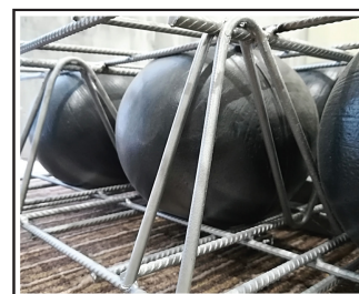
■ LATTICE GIRDER IN BUBBLEDECK CAST-IN-SITU SYSTEM
