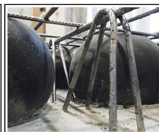
■ LATTICE GIRDER IN BUBBLEDECK PRECAST SYSTEM
